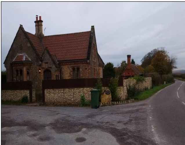
Enclosure including gabion wall with fence above – October 2017
